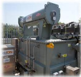
The FCL instantly suppresses excessive current and recovers to normal load promptly upon fault clearance - being always ready for consecutive short circuit events. The FCL increases network capacity and improves grid resilience and reliability, while significantly lowering capital expenditures and operating costs. The FCL is reliable and robust, and is easy to install and maintain.
